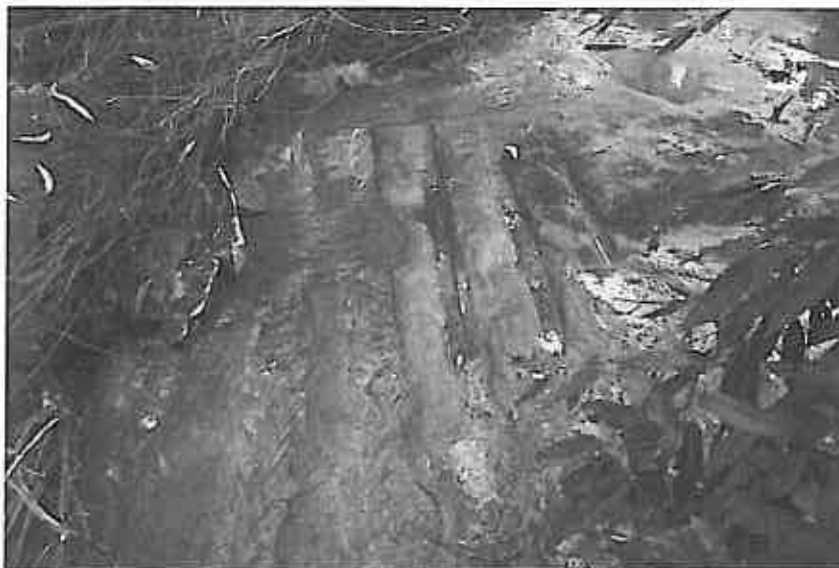
Plate 16: Damage to rock platform from grader and assumed to date from F3 construction
